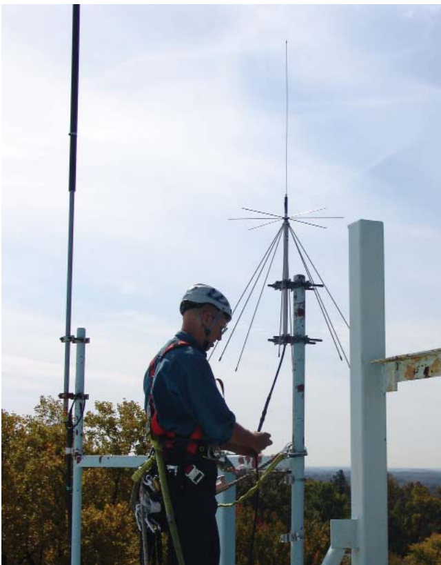
Mike, W3MC installing discone
