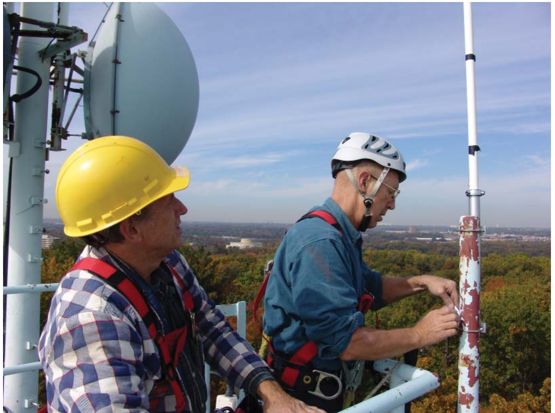
Jim, WI3N and Mike, W3MC installing new antenna
